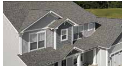
ROOFING AND VENTILATION
